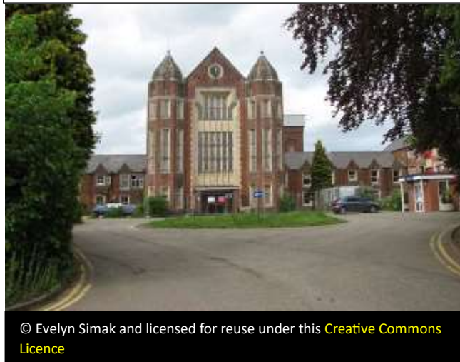
The former St Michael's Hospital in Aylsham in 2009
