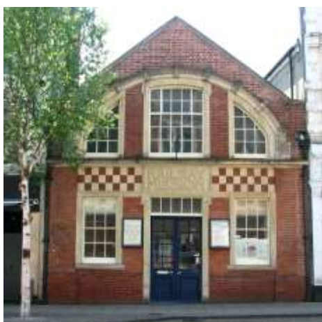
© Evelyn Simak and licensed for reuse under this Creative Commons Licence
