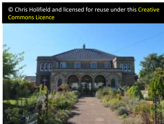
Former Congregational church in Bungay, now Emmanuel, a combined Methodist and URC
