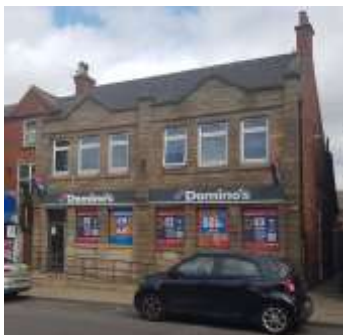
Domino's at 21 Station Street in August 2023
