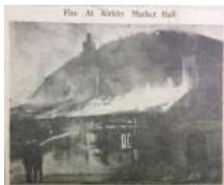
Fire at Market Hall 1947. Source KIAP
