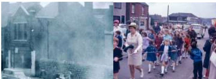
Above left – close up of 2 Station Street. Source KLM Above right – this image from late seventies clearly shows that number 2 had already been demolished. Source Alwyn Bowskill
