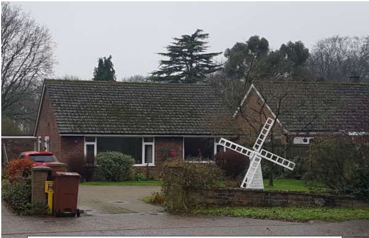
166 Drayton High Road in December 2021 showing the windmill in the front garden
