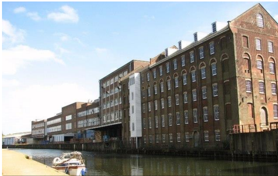
© Evelyn Simak and licensed for reuse under this Creative Commons Licence
