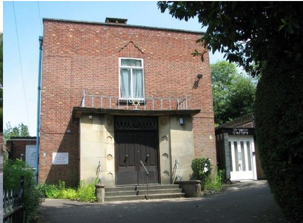
© Evelyn Simak and licensed for reuse under this Creative Commons Licence
