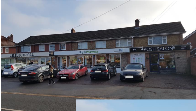
Row of shops on Middletons Lane between Links Avenue and Reepham Road
